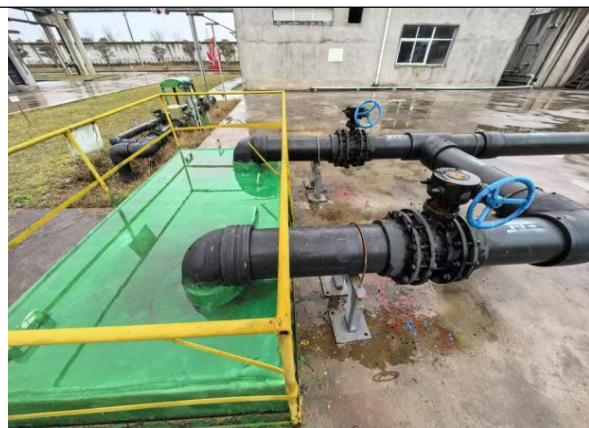
封闭池口并加装尾气管
